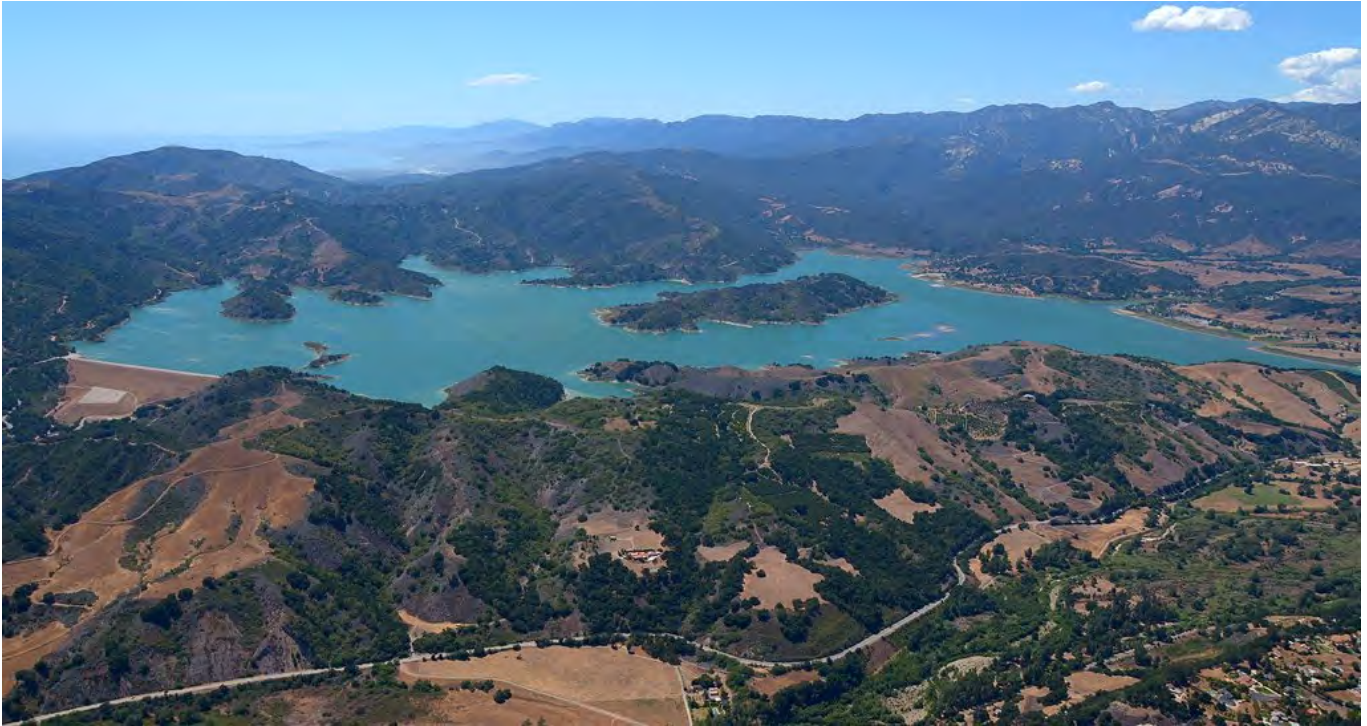
FIGURE 4-2 LAKE CASITAS AND CASITAS DAM
